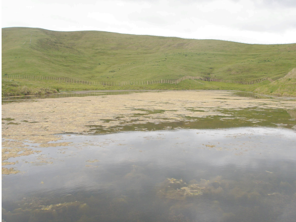
Dam in September 2011 (first application on 21 November 2011).
